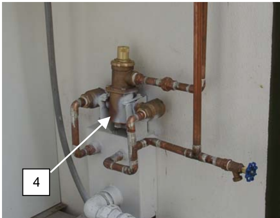
Mixer Valve With Fabricated Mount
